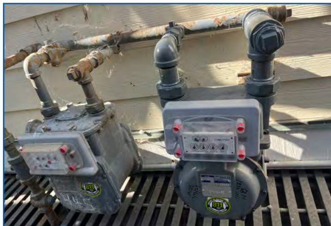
New meter installation
